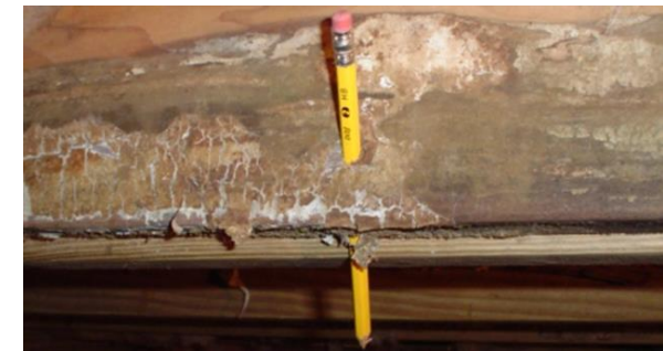
Degradation of cell-wall carbohydrates and cavity formation by brown-rot and soft-rot in wood
